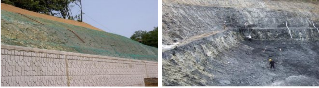
(사진 8-12) 쏘일네일링(soil nailing)
