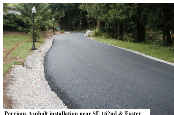
Pervious Asphalt installation near SE 162nd & Foster
